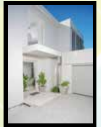
Basement to Roof
